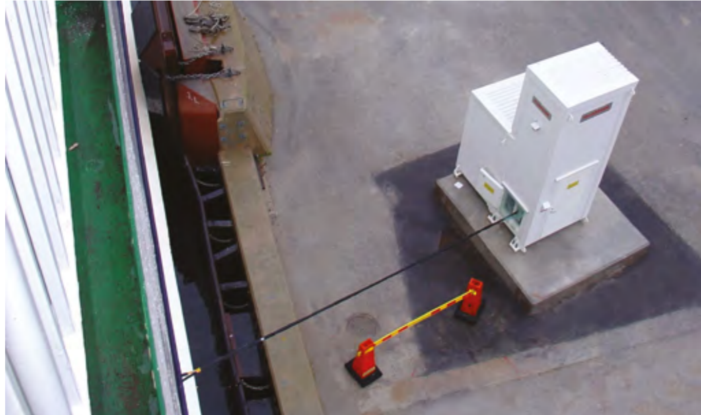
MOOREX® mooring rope angles are always optimal, rope forces remain high, and the ship's position is accurately maintained. Compact MOOREX® ashore units save space onboard.
