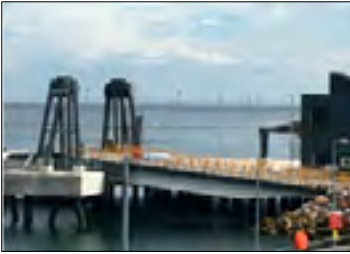
2017 Linkspan Brodick, United Kingdom Caledonian Maritime Assets Ltd
