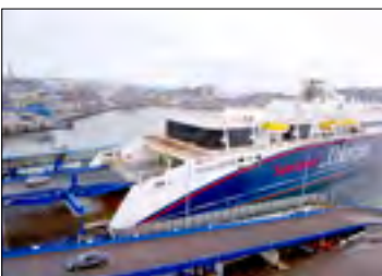
2007 Linkspan, two-tier ramp system Kristiansand, Norway Color Line AS
