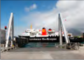
2011 Linkspan, conversion Port Askaig, United Kingdom Argyll & Bute Council
