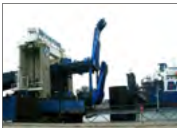
2002 Two-tier linkspan, conversion Dunkerque, France Port of Dunkerque
