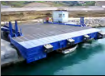
2009 Two linkspans Tanger, Morocco Tanger Med. Port Authority (TMSA) SRPTM
