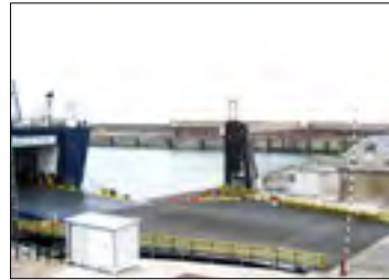
2009 Linkspan Rosslare, Ireland Irish Rail BAM Contractors
