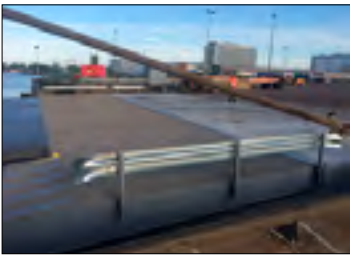
2015 Linkspan Gothenburg, Sweden Port of Gothenburg
