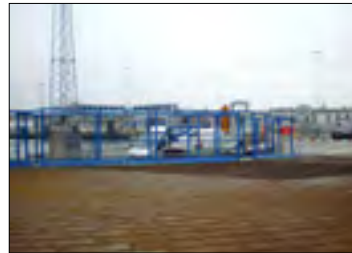
2008 Passenger gangway, conversion of pontoon Ystad Hamn, Sweden Ystad Hamn AB
