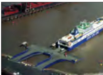
2006 Linkspan, floating Immingham, United Kingdom DFDS/ABP
