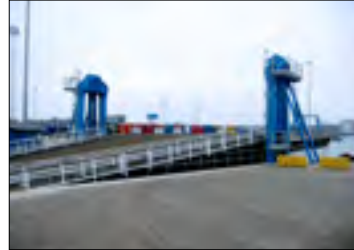
2004 Linkspan Ipswich, United Kingdom Associated British Ports (ABP)
