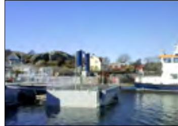
2013 Water Taxi Terminal Öckerö, Sweden The Municipality of Öckerö
