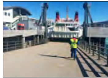
2015 Linkspan Ullapool, United Kingdom Caledonian Maritime Assets Ltd
