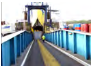
2006 Linkspan, conversion Newhaven, United Kingdom Port of Newhaven
