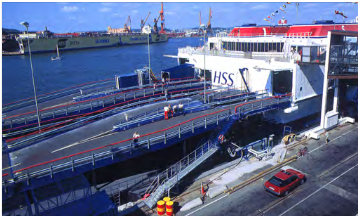
Linkspans for high-speed ferry HSS 900 Stena Carisma, Gothenburg, Sweden, 1997
