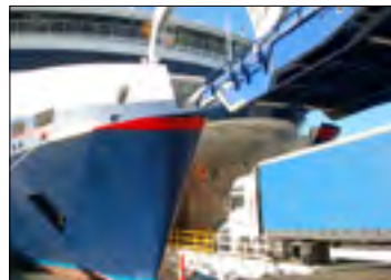
2008 & 2007 Linkspans, two-tier ramp system Hirtshals, Denmark Color Line AS
