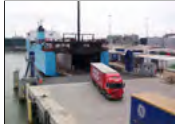
2007 & 2006 Linkspan Vulcaanhaven, Rotterdam, The Netherlands Norfolkline BV
