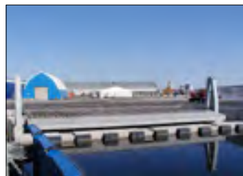
2006 Linkspan Sundsvall, Sweden Port of Sundsvall
